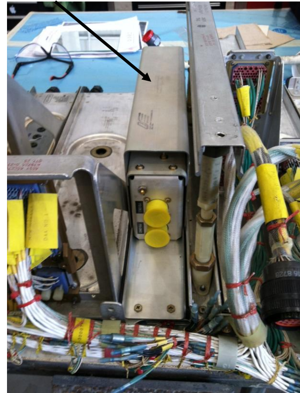
New synchro Chassis in EE bay
